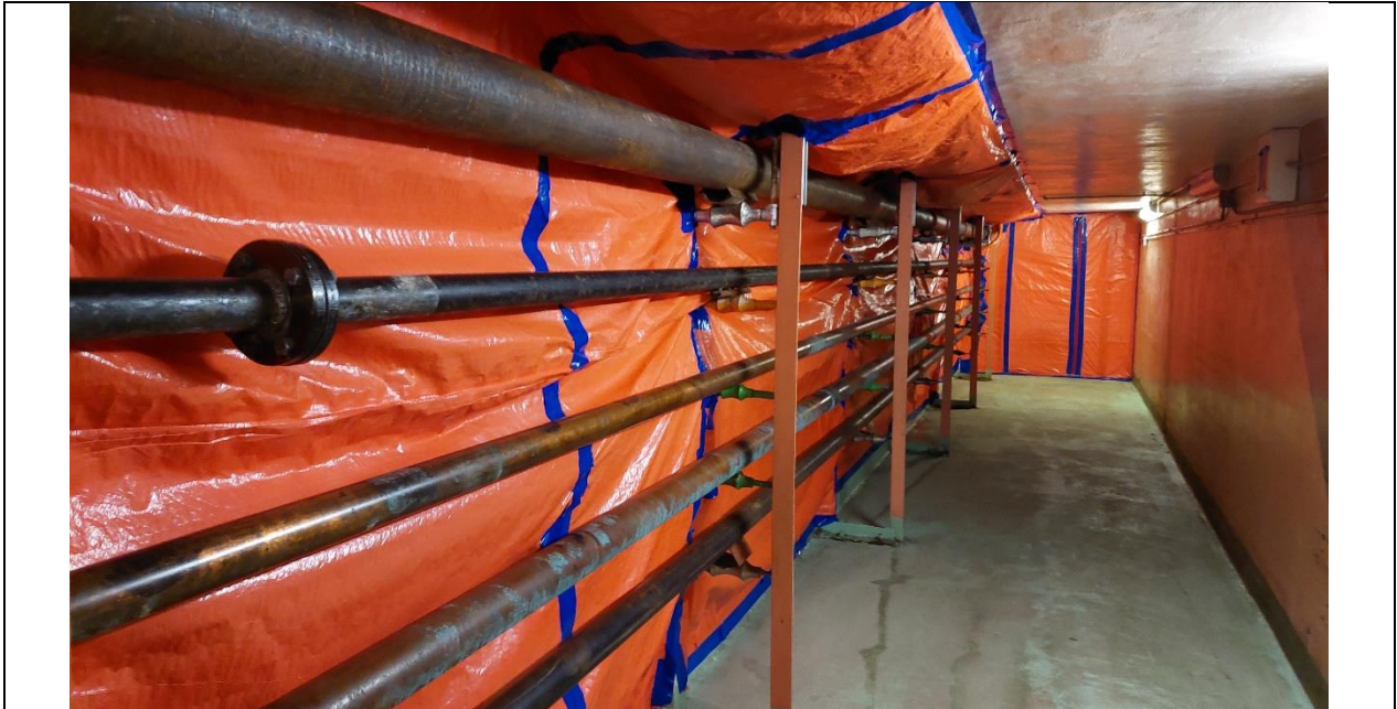
Picture 1 – Avon Crest Tunnel
